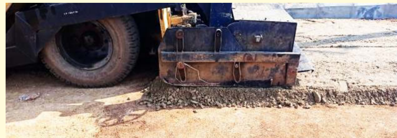
Heavy Duty Road Laying for Extra Durability and Long Life
