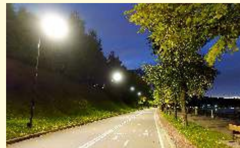
Street Lights Lining the Roads
